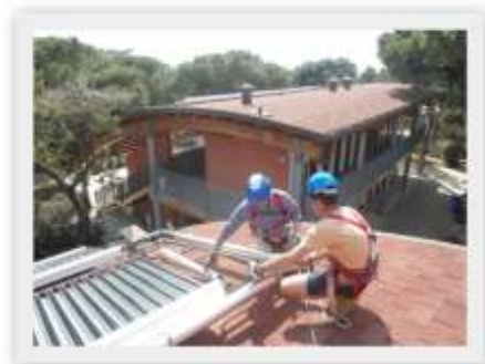
INSTALLING SOLAR PANELS
